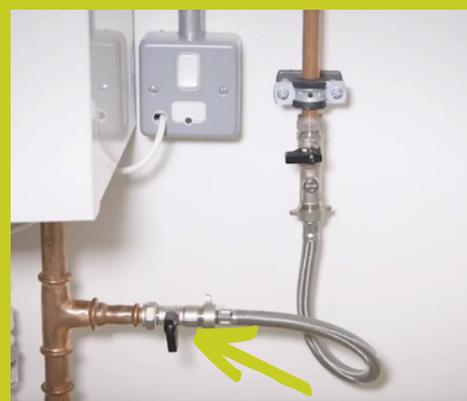
Tap to boiler **slowly** open to allow water into the heating system.
