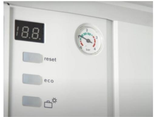
**Do not overfill the pressure past 1.5 bar on the gauge as it could damage the boiler and system.**
